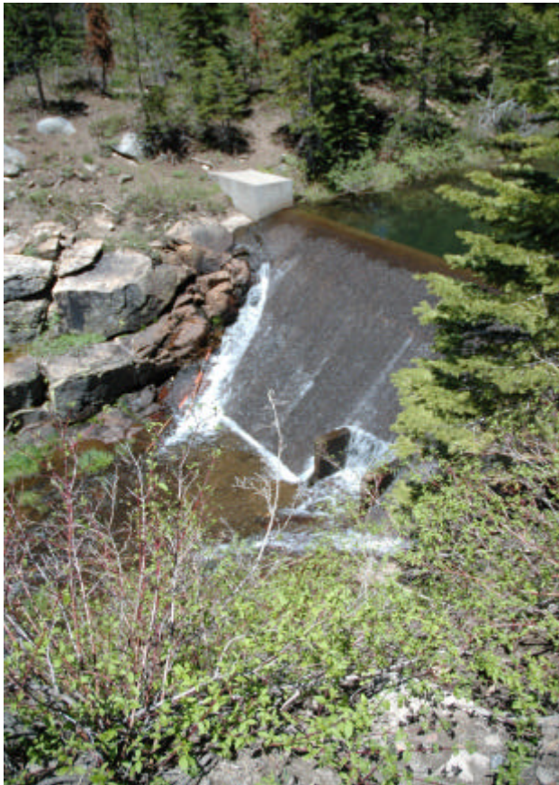
Serena Creek Spillway
